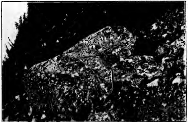
PICKING ON A "BENCH" TO LOOSEN GOLD-BEARING GRAVEL FOR THE SLUICES BELOW.
